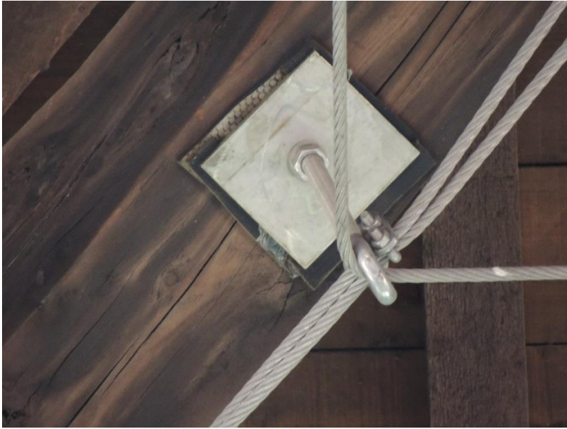
Figure 3. A detail of the wood beam reinforcement of the roof of one tower of Pavia Castle, Italy. The new addition is completely reversible. Project: Lorenzo Jurina (photo: Andrea L'Erario, 2014)
